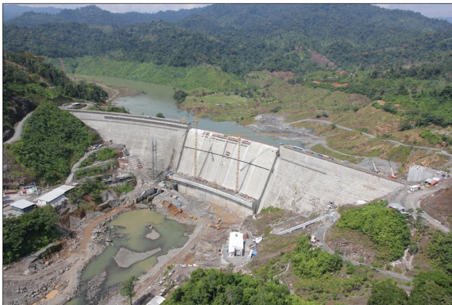
Figure 1: Changuinola 1 Dam, Panama
