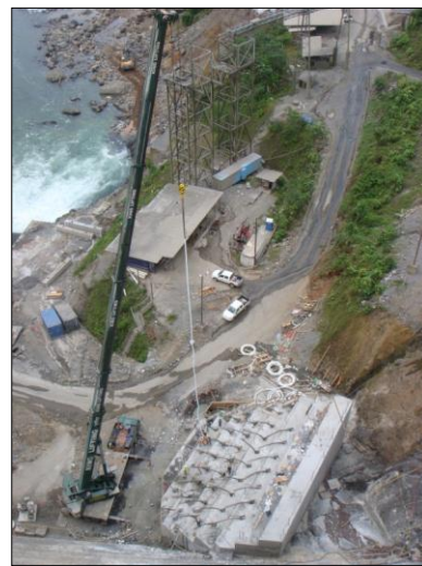
Figure 10: Installing anchor cables
