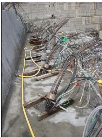
Figure 9: Anchor cables installed
