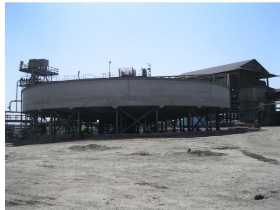
Figure 4: Kamoto Copper Mine Process Plant, DRC
